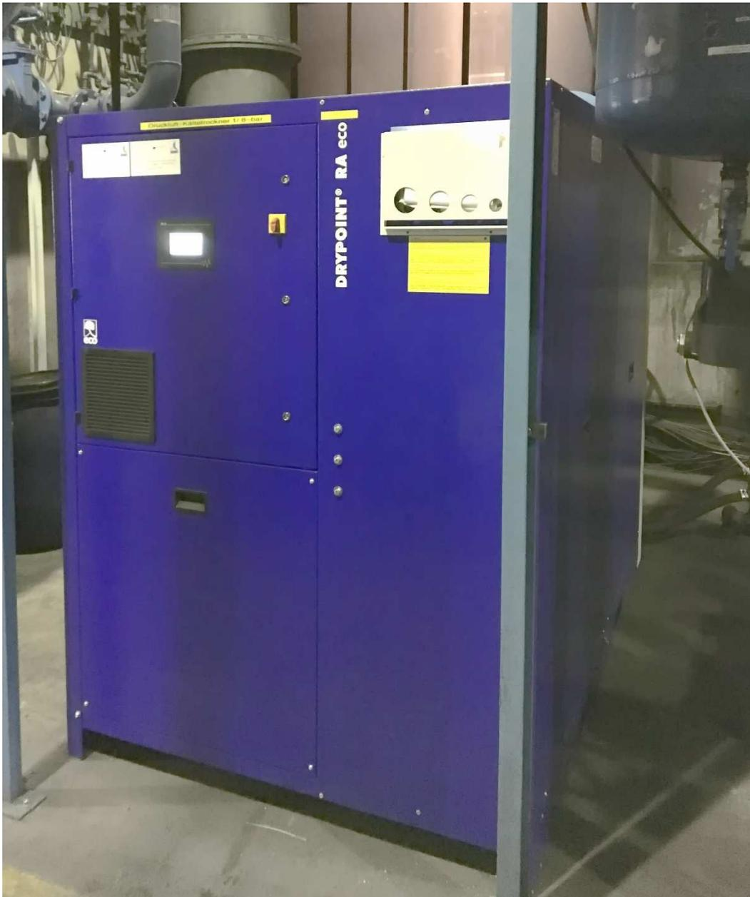
For volume flows from 1000 m<sup>3</sup> per hour upwards, the DRYPOINT RA eco combines frequency control of the refrigeration compressor with cycling operation. At these high output rates, the fan is also frequency-controlled, resulting in optimized dryer performance combined with lowest possible energy consumption. This control logic also ensures that the units can be switched within seconds from high to low delivery and vice versa.
