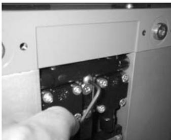
6. Replace and tighten purge plug fixing screw in upper valve block.
